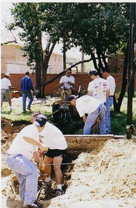
The brothers of Eta Upsilon Chapter at the University of Texas-Arlington dig up and replace an old sewage line.
